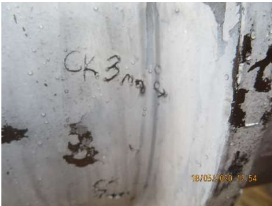
PHOTOGRAPH NO. 8 - 3mm crack detected
